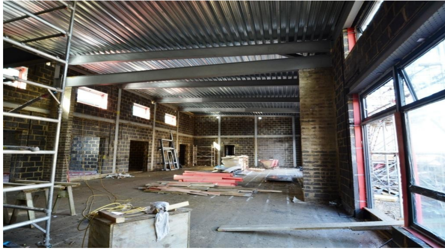
A view down the new hall.
